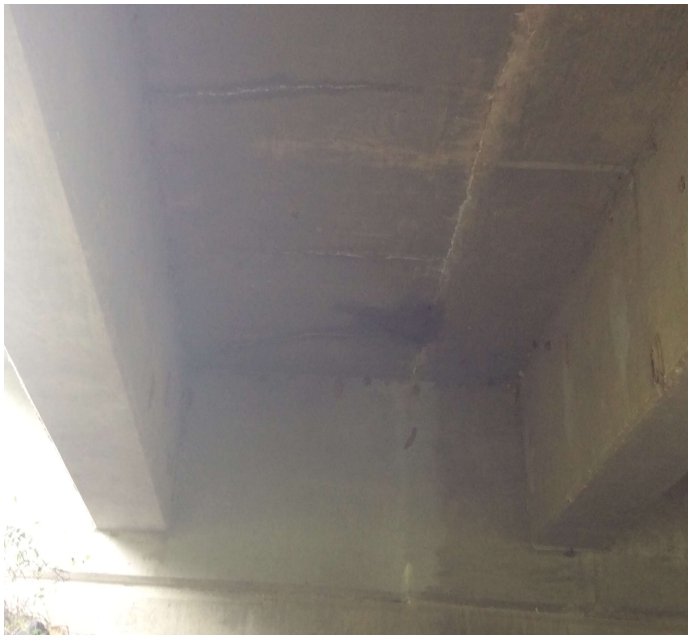
PHOTO 1 Description Soffit, Span 7 near bent 8 between girders 1 & 2 the soffit has moisture seeping from the deck at the construction joint.
