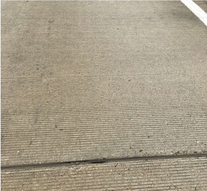
PHOTO 2 Description Deck - Span 5: Cracking
