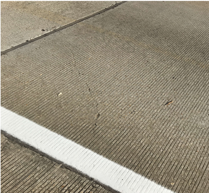
PHOTO 3 Description Deck - Span 7: Cracking
