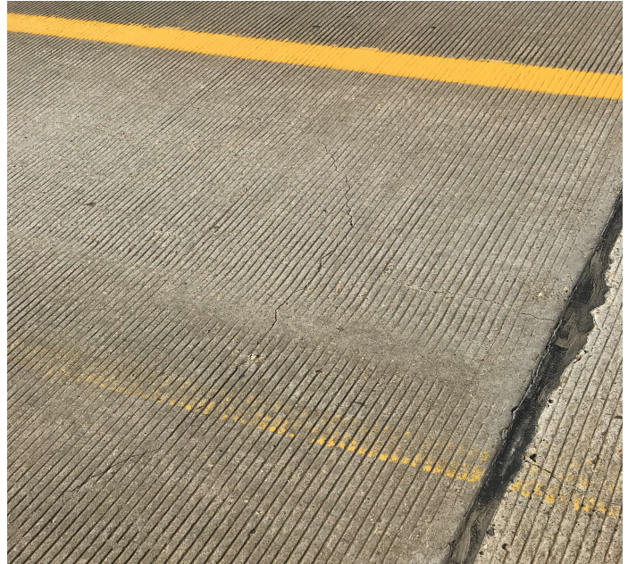
PHOTO 4 Description Deck - Span 7: Cracking
