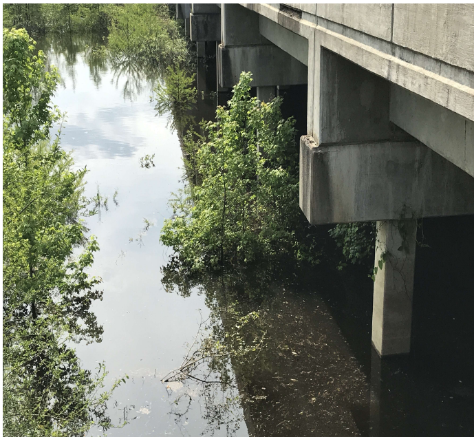
PHOTO 1 Description End-slope - Span 6 right : Vegetation
