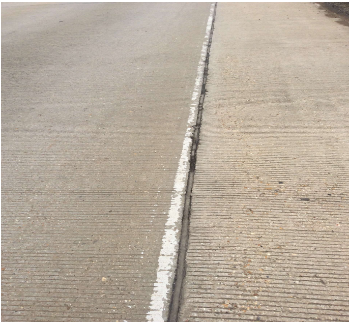
PHOTO 2 Description Deck joint at soffit crack, joint material has lost bond allowing moisture to seep through deck. ( See soffit photo).
