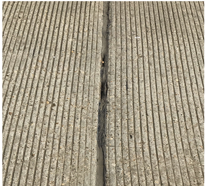
PHOTO 1 Description Joint - Bent 2 : Loss of adhesion
