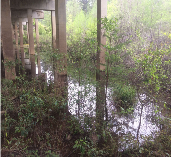
PHOTO 3 Description Span 2 trees growing under the bridge. Common all spans.
